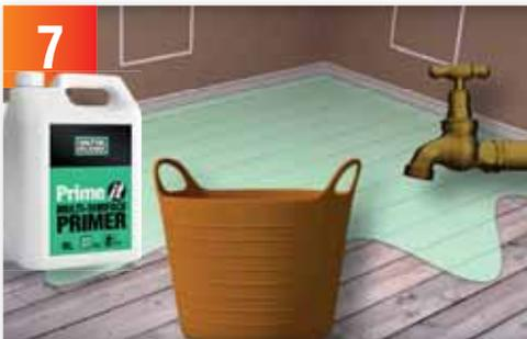
Whilst the primer on the boards is drying commence with priming of the substrate using UltraFloor Prime-IT MSP. The primer should be diluted 3 parts water to 1 part primer and allowed to fully dry.
