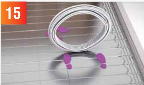
Above picture: illustration purposes only, ideally the pipe should be unrolled using a de-coiler or in the horizontal position to allow for ease of laying the pipe (This will stop the pipe trying to spring out of the boards at the end of the panels).
