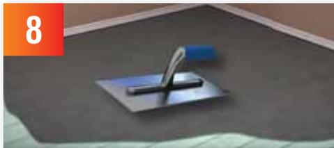
Apply UltraTile Proflex S2 adhesive to the subfloor using a notched trowel to give a minimum 3mm adhesive bed. Laying the boards as you go (The depth of the adhesive bed may need to increase if the substrate is not sufficiently level. Additional levelling compound may be needed if areas are any deeper than 2-3mm).
