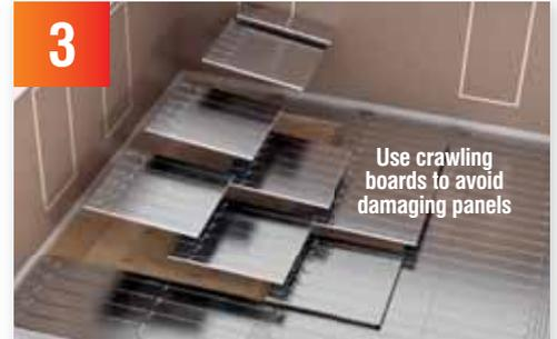
3 Lay the boards across the floor with the grooves facing upwards, making sure the pipework runs are calculated correctly to reach manifold position.
