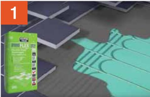
**1** Fix the tiles using UltraTile ProFlex S2 adhesive. Ensure that every pipe channel and void surrounding the pipe is fully encapsulated with tile adhesive.
