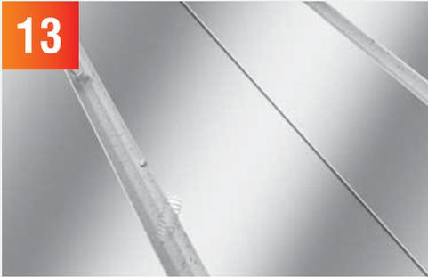
Ensure your floor is free from any debris before installing the pipe. It is important to check in all the grooves as the pipes could be damaged during installation if there are any obstructions.
