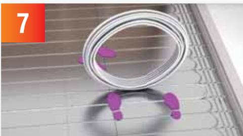
7 Above picture: illustration purposes only, ideally the pipe should be unrolled using a de-coiler or in the horizontal position to allow for ease of laying the pipe (This will stop the pipe trying to spring out of the boards at the end of the panels).
