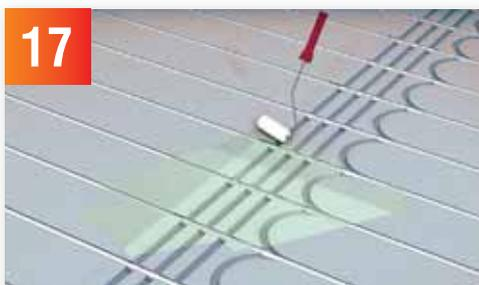
Prime the upper face of the boards with a neat coating of Ultra Prime-IT MSP bonding primer. This should be applied by brush or roller in a thin film. Allow to thoroughly dry to a clear green film, (approx 1-4 hours).
