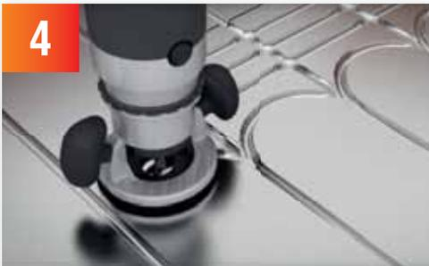
4 You may be required to modify the heating panel to navigate around permanent fixtures. If you find you need to create a new channel then this can be done with a knife or router.
