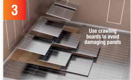
Loose lay the boards across the floor and number the boards on the upper face to identify position of each board, making sure the pipework runs are calculated correctly to reach manifold position.
