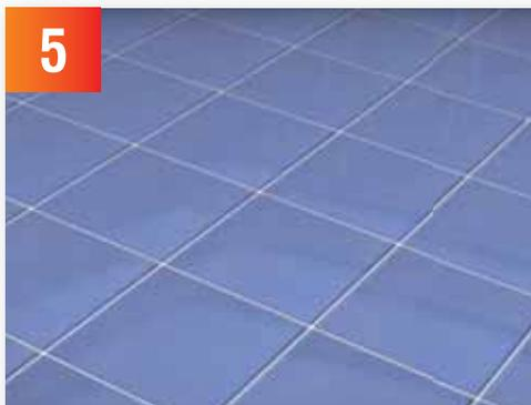
Grout the tiles using UltraTile Flex Joint grout. Allow to fully cure before trafficking.
